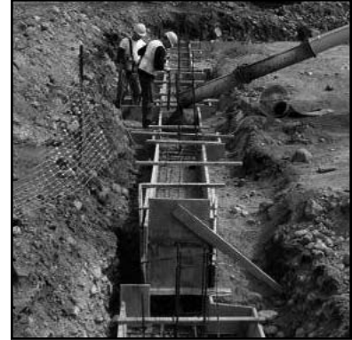
April 2014 Concrete is poured for the footings
